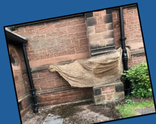
Matching the mortar of the brickwork for re-pointing
