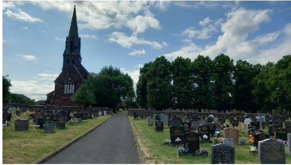
View of building from Whitby's Lane gate
