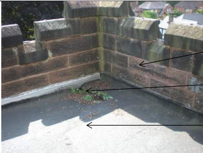
Photograph 1 Tower Roof SE Corner – Low / Rainwater Outlet
