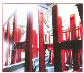
Above: An image showing a partly installed, new "H" pattern bellframe.
