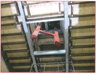
Above: An image of a 'H' frameside passing through a floor that our bellhangers have recently built.
