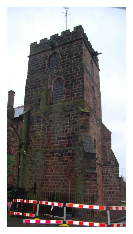
This wall contains louvre window openings at belfry and clock chamber levels. To the north east corner, there is a small projection which houses the spiral staircase and extends up to clock chamber level. There are two small window openings towards the top of this projection which give light to the staircase. Again, the masonry appears to be in generally fair condition, consistent with its age, with no evidence of any significant cracking, recent or ongoing movement.
