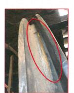
Above: Images showing the condition of the bell wheels, including: Split spokes, burst feather fillets, replacement shrouding, and worn soling.
