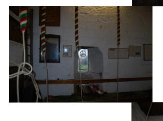
The walls at this level are partially obscured by timber panelling. Where they are exposed, they have been painted. There does not appear to be evidence of any significant cracking, recent or ongoing movement to the masonry.
