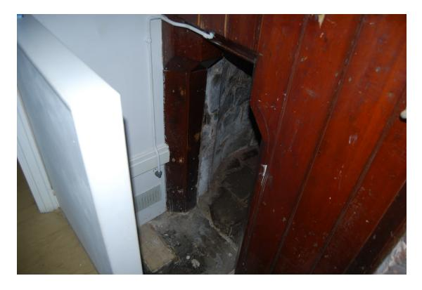
The original floor level has been raised to match the nave floor level. Toilets and a central heating boiler have been installed relatively recently. The walls, where exposed, have been painted and the masonry appears to be in generally fair condition, consistent with their age, with no evidence of any significant cracking, recent or ongoing movement.
