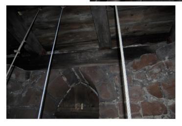
The walls at this level are of exposed stone masonry construction. There are what appear to be the beginnings of squinch arches below belfry floor level, the purposes of which are unknown. Possibly there was some intention of building a spire at some time in the past. There does not appear to be any evidence of significant cracking, recent or ongoing movement to the masonry.
