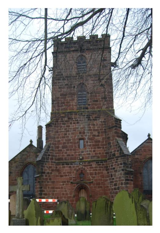
This wall contains louvre window openings at belfry and clock chamber levels, a small, glazed window opening giving light to the ringing chamber and a door opening at ground level with a small quatrefoil window immediately above this. Again, the masonry appears to be in generally fair condition, consistent with its age, with no evidence of any significant cracking, recent or ongoing movement.
