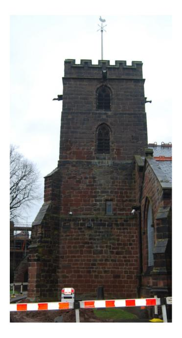
This wall contains louvre window openings at belfry and clock chamber levels and a small, glazed window opening giving light to the ringing chamber. The masonry appears to be in generally fair condition, consistent with its age, with no evidence of any significant cracking, recent or ongoing movement.
