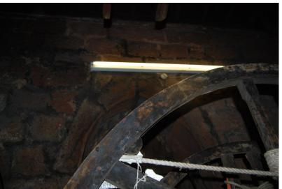
The walls at this level are of exposed stone masonry construction and, where they are not obscured by the bell frame, the masonry appears to be in fair condition, consistent with its age, with no evidence of any significant cracking, recent or ongoing movement or other structural distress.
