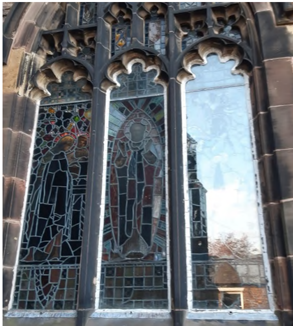
2. Christopher Whall window: protection fully mortared in (and cracking).
