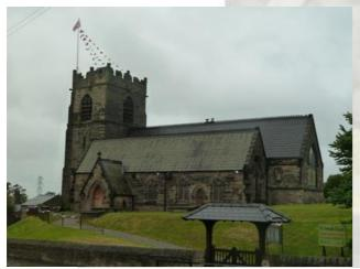
The church is built from coursed and squared rubble in large blocks with a roof of Westmorland slate with ridge cresting. Its plan consists of a west tower, a nave, north and south aisles with gable roofs, a south porch, and a chancel. Heraldic shields over the west door date it between 1504 and 1521. The tower is in three stages with angle buttresses and an embattled parapet.
