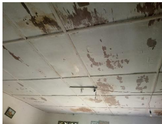
Internal view dampness to ceilings
