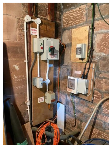
Photo 5.3 Electrical supply to organ air compressor
