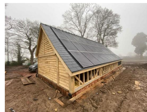
Photo 8.2 59m 2 array on log store in Shropshire
