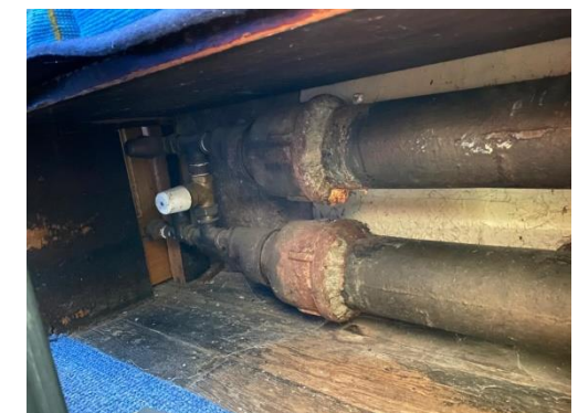
Photo 4.5 Caulked joints on cast iron pipework
