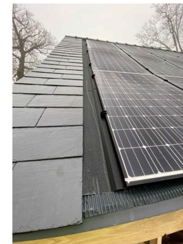
Photo 8.3 PV panels are recessed into a tray in the roof
