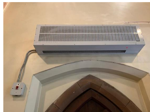
Photo 4.8 Electric over door heater
