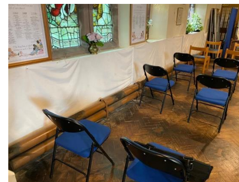
Photo 4.4 Cast iron heating pipework
