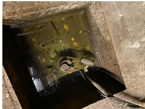
Photo 4.11 Sump and pump in cellar
