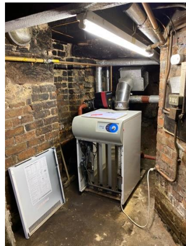
Photo 4.1 Existing Ideal Concord gas-fired boiler in cellar
