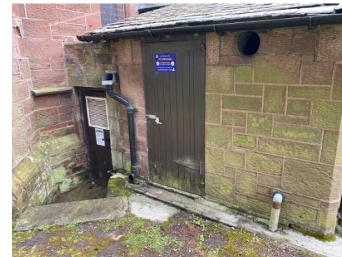
Photo 4.2 Ventilation to the cellar is via a grille in the door outside
