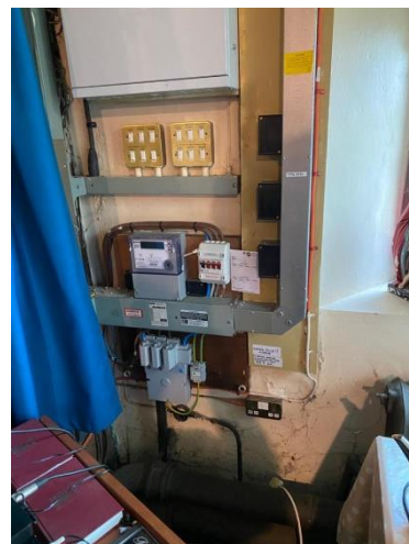
Photo 3.1 Incoming electricity service head and meter
