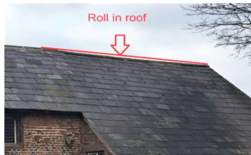
Figure 2: Alignment of roof demonstrating "Roll" within roof covering.
