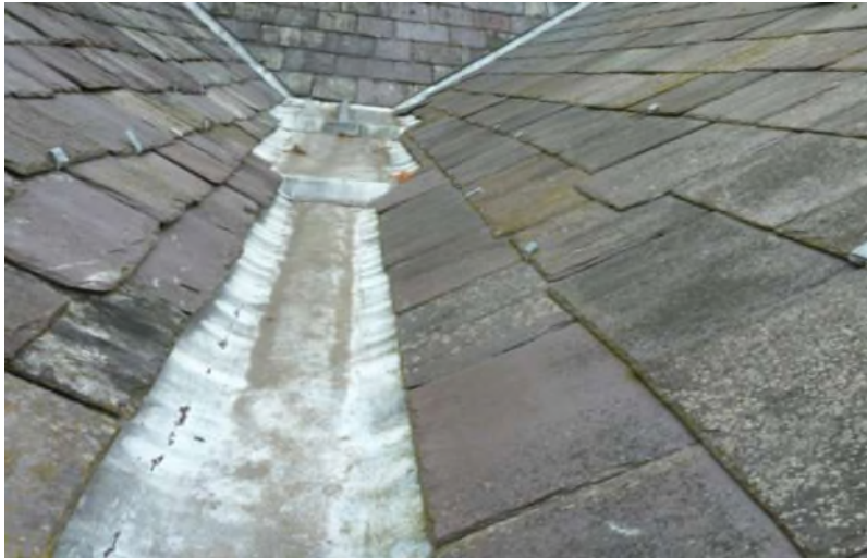
Figure 3a: External view of lead gutter and slates fixed with “tingles”
