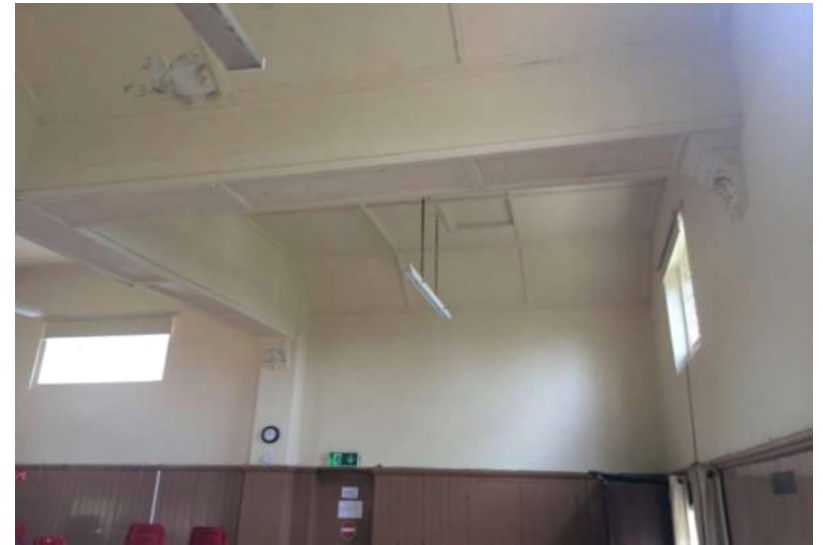
Figure 3b: Interior view of water damage under lead central gutter.
