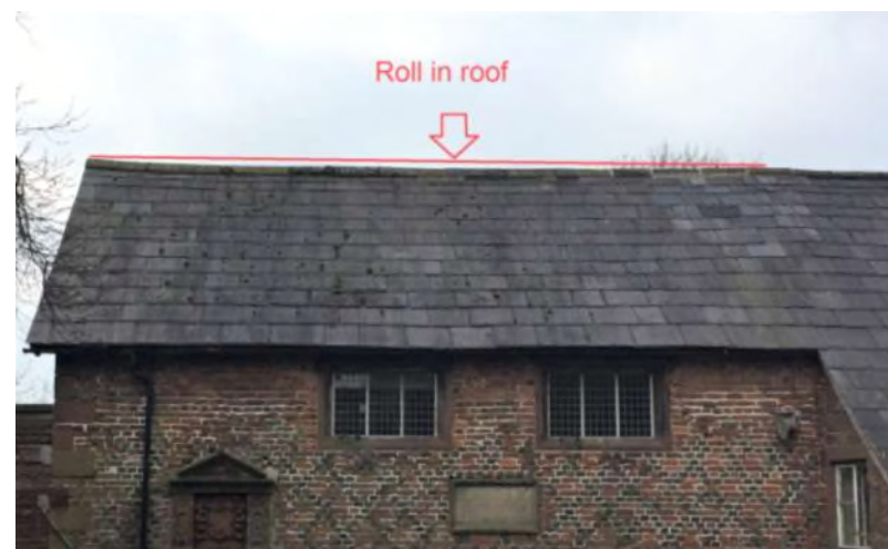
Figure 1: Alignment of roof demonstrating "Roll" within roof covering.
