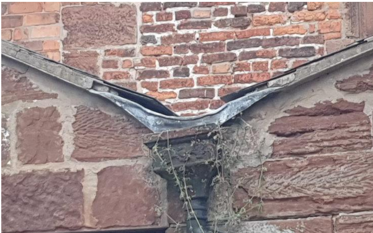
Plate 12: Drainpipes and gaps in the roof of B1 .
