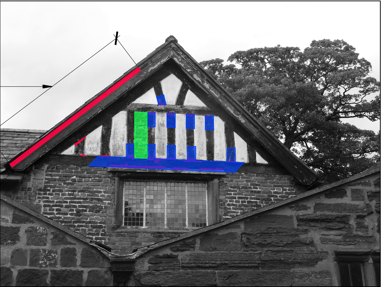
TIMBER FRAMING TO GABLE – SOUTH FACING ELEVATION
