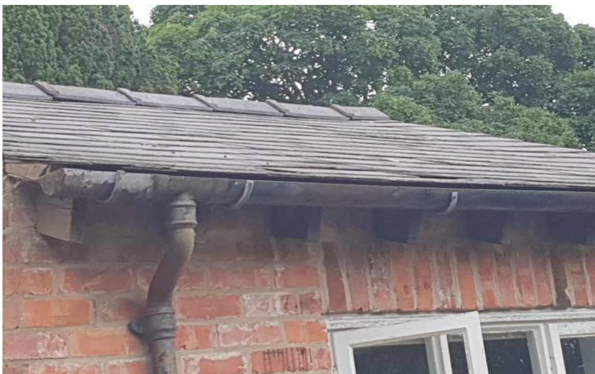
Plate 6: Some of the lifted slate and ridge tiles on B1 .
